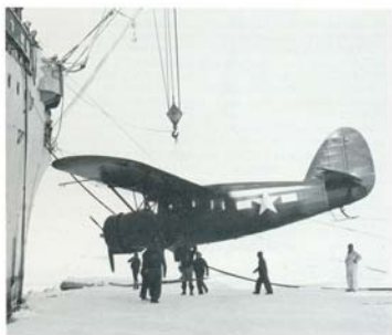
J2F-6 Duck seaplane, attached to the US Coast Guard icebreaker NORTHWIND during Antarctic OPERATION HIGH JUMP of 1946-47. Aircraft is painted overall Aluminum varnish with a Flat Black anti-glare panel forward of the windscreen. Coast Guard insignia is carried on the forward section of fuselage just above bottom wing leading edge. (USCG)
